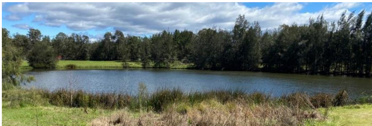
Figure 6: Existing dam intercepting runoff from the site, prior to discharging to the Sydney International Regatta Centre.
